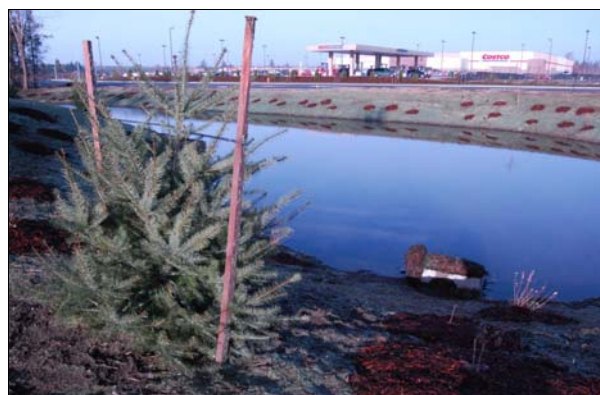
A stormwater runoff pond built near the new Costco store.
